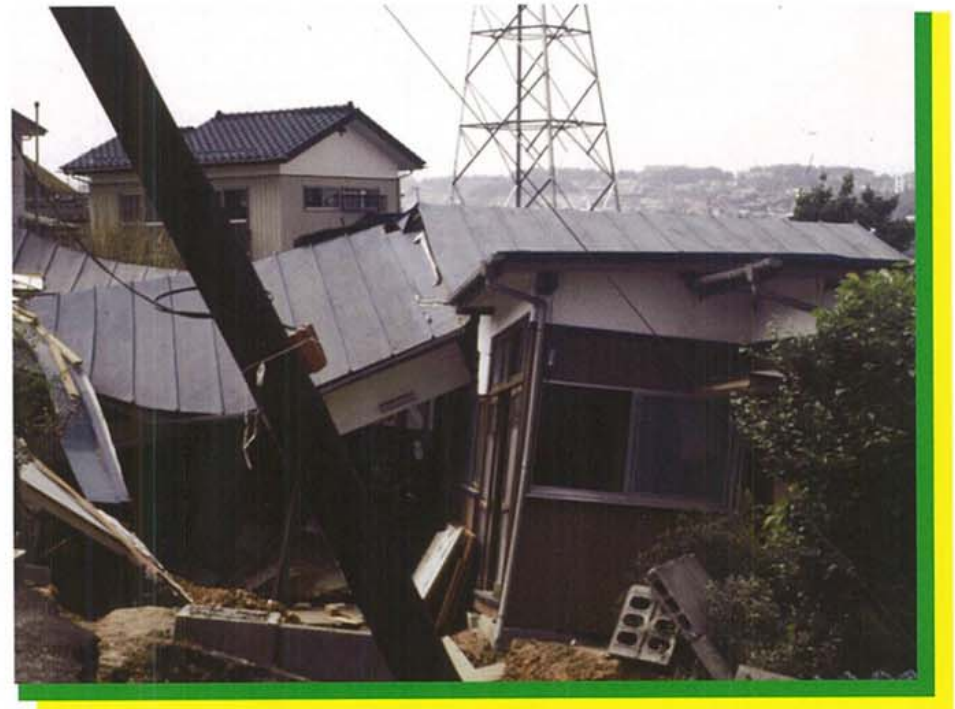
Damaged buildings following the Miyagi-oki earthquake of June 12, 1978
