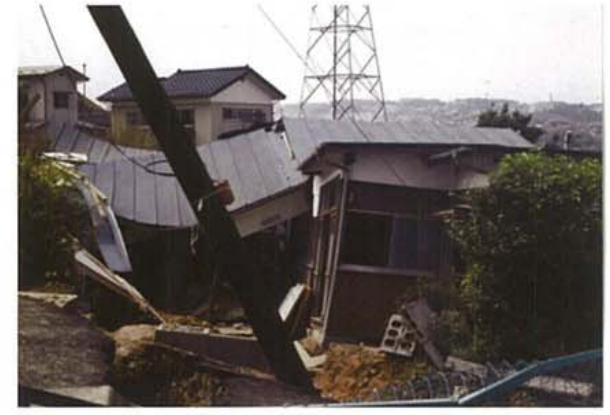
1978 Miyagi-oki earthquake (Midorigaoka, Sendai City)
