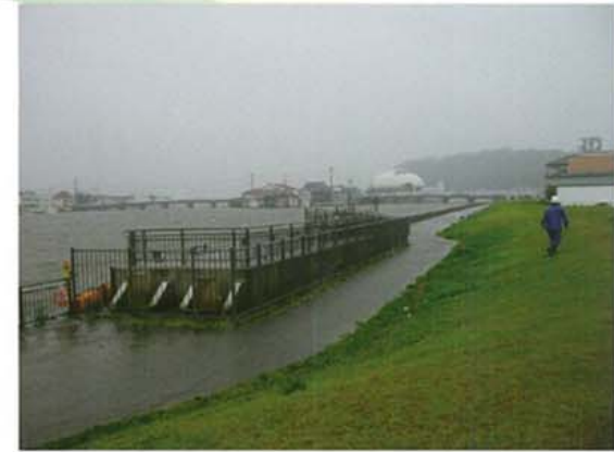
Swelling and flooding at Kitakami River caused by typhoon
