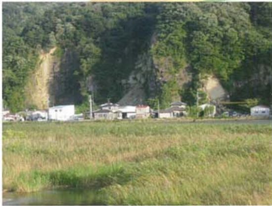
Landslides along sloping land↑ Photograph on right: Destruction in vicinity →
