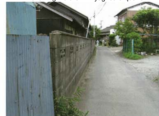
Will the concrete block walls and evacuation routes survive an earthquake?
