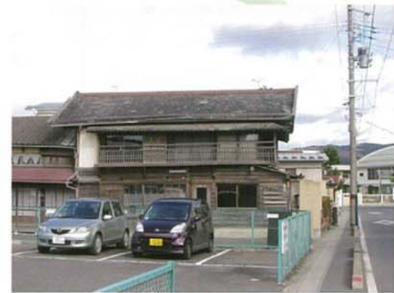
Old residential buildings and transformers
